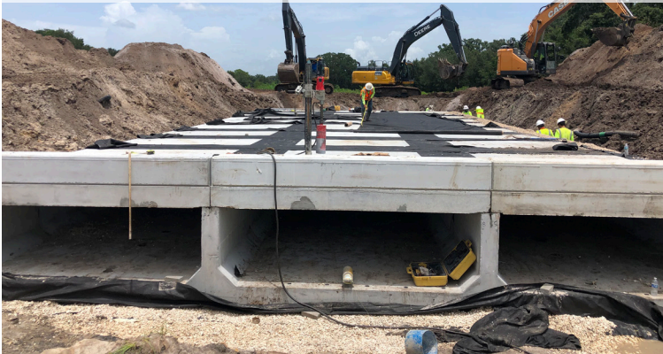
Bridge Box Culvert Installation
