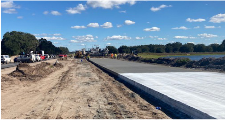
Concrete Paving Operations
