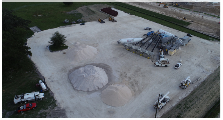
Portable Concrete Batch Plant
