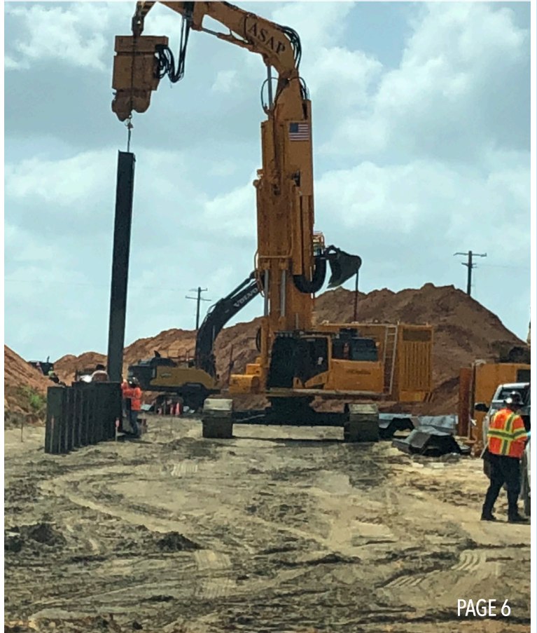
Driving Sheet Pile
