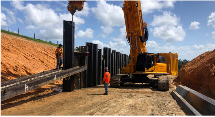
Sheet Pile Installation
