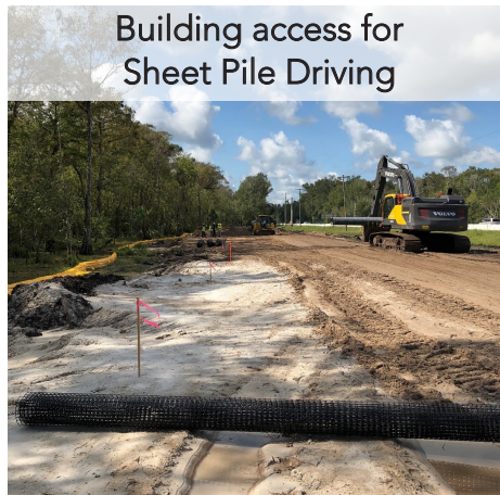
Subsoil Excavation
