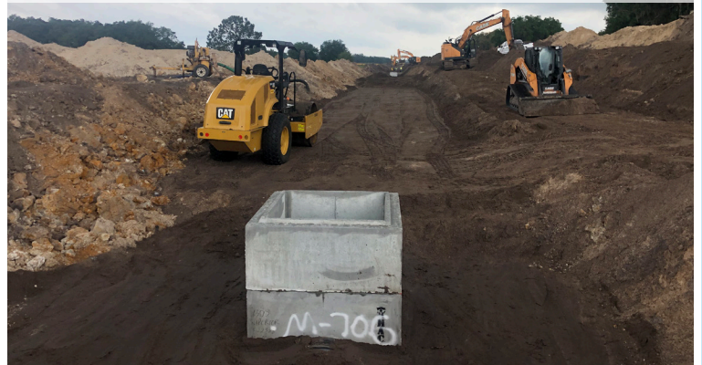
Storm Sewer Installation
