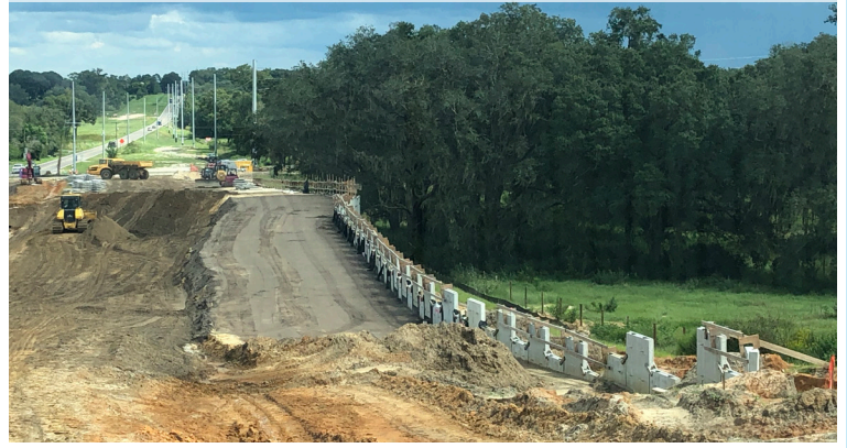
MSE Wall Installation
