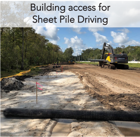
Subsoil Excavation
