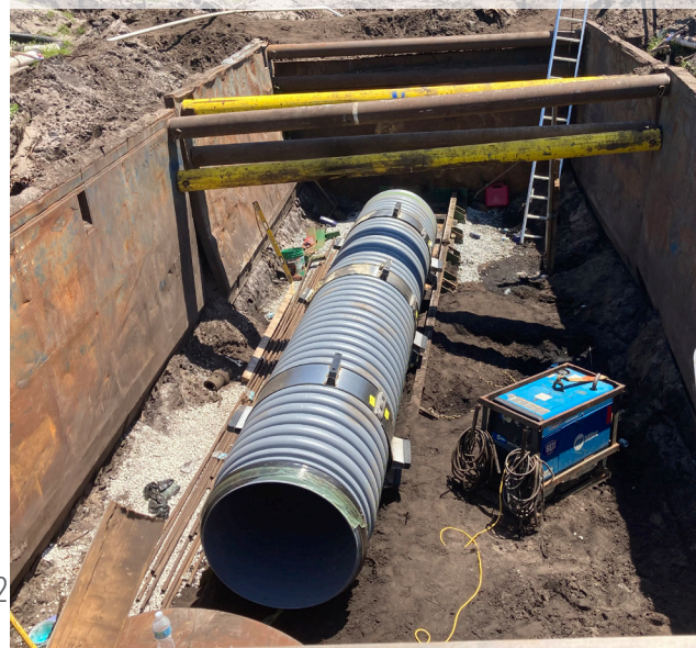
36-in Storm Drain Placed Inside 54-in Jack and Bore
