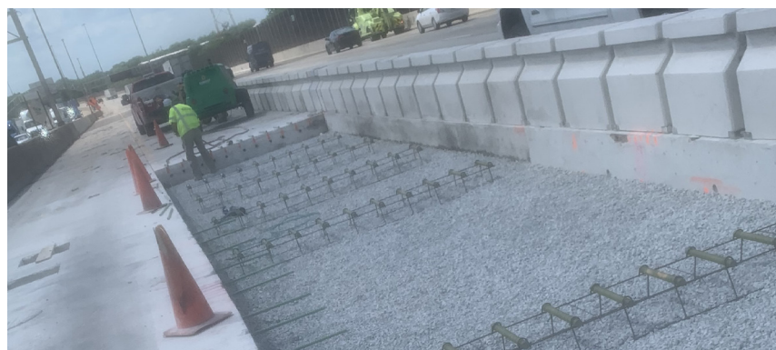
90' of PCCP for the weigh-in-motion (WIM) station
