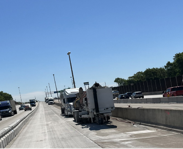
Profile grinding and longitudinal grooving completed
